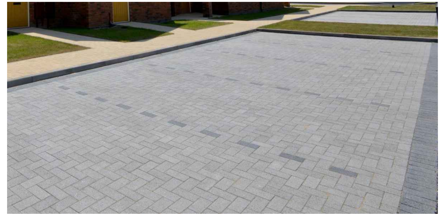
PAVING TYPE A (PARKING AND ROAD SURFACING) PARKING BAYS DEFINED WITH LIGHTER COLOURED BLOCK
